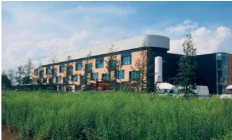
View of the new building from the south-east with the container docking station (by the black wall).
